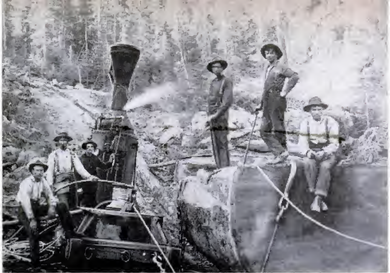
Donkey steam engine was the workhorse. Mounted on skids, it reeled in cable to pull itself up the mountains
